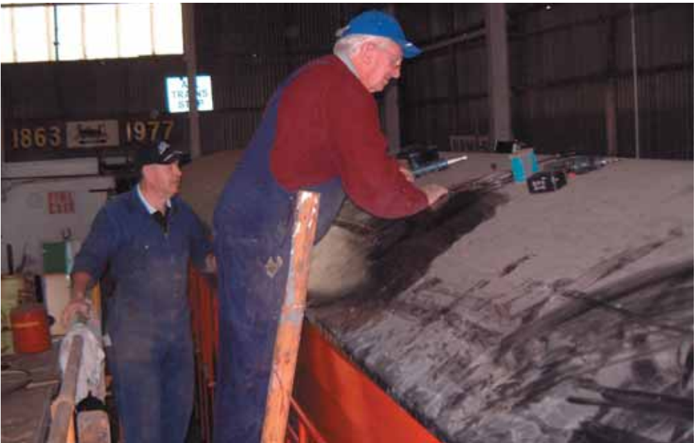
Keith Brown and Graham Inwood placing the roof ventilators on 'A1177'.
