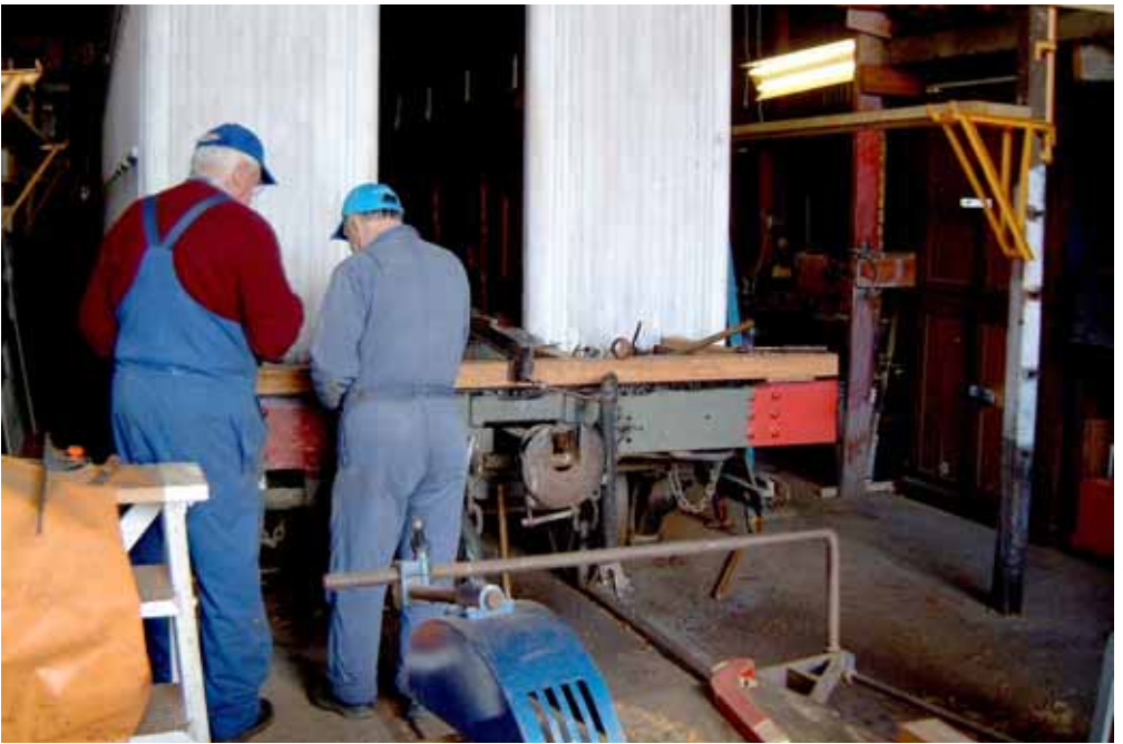
Keith Brown and Graham Inwood preparing the end decking of 'A1177'.
