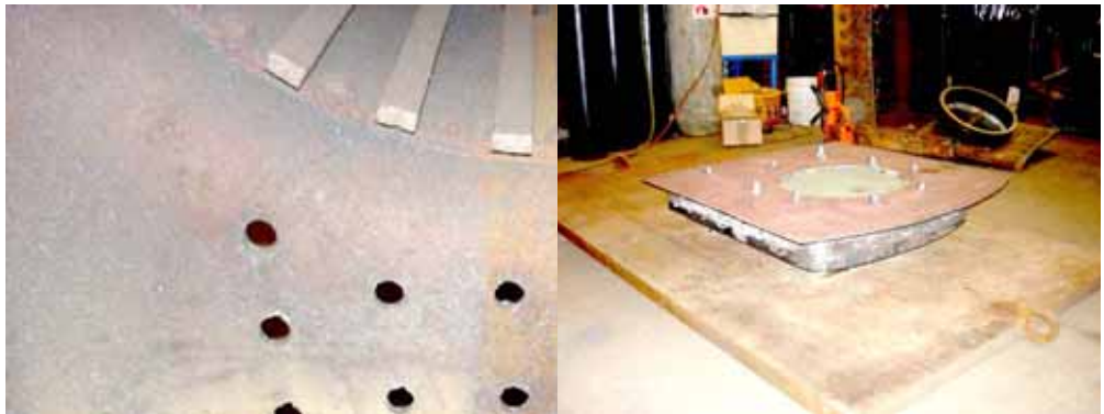
Left; Showing major renewals in the foundation ring corners.
