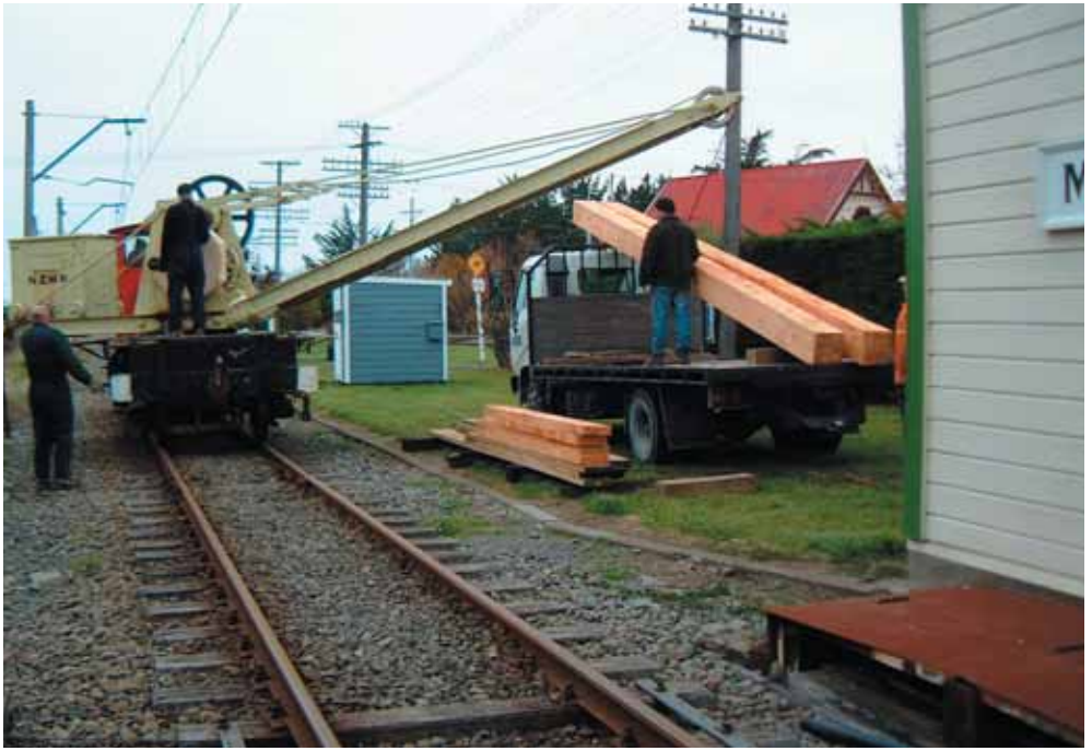
Unloading new Macrocarpa signal posts. 12" x 12" and seriously heavy!
