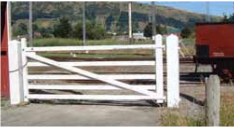
Finally, the gate is fitted.
