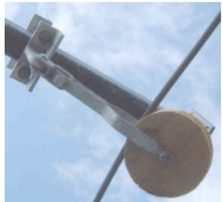
Changing the carrier and detail of the home made feeder pulley carrier.
