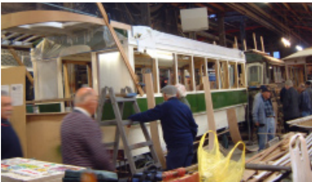
Members inspecting the restoration of a tram car body.
