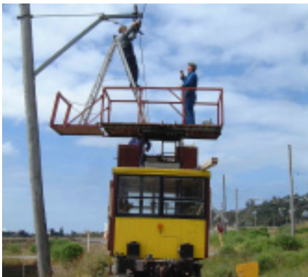
Changing the carrier and detail of the home made feeder pulley carrier.
