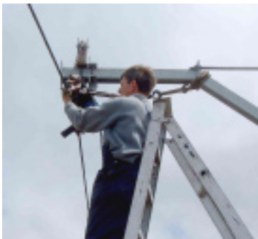
Changing the support and the platform raising mechanism .
