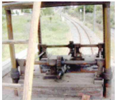
Changing the support and the platform raising mechanism .
